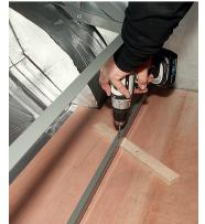
Check once again that the lower support frame is straight and true. Using some offcuts of wood, lift the lower framework up slightly and slide the offcuts under so you can drill pilot holes for the self-tappers that will secure the frame to the ply floor. As per the instructions, fit one either side of the frame
