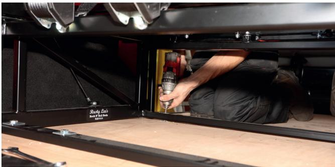
**17** For added piece of mind, and to ensure the bed sat perfectly level, two further holes were drilled through the front rail of the bed. The one closest to the wheelarch fell 170mm from the 'arch, in a double-skinned section just between the spring and chassis rail underneath, so you may have to drill at a slight angle here. Measure twice and drill once
